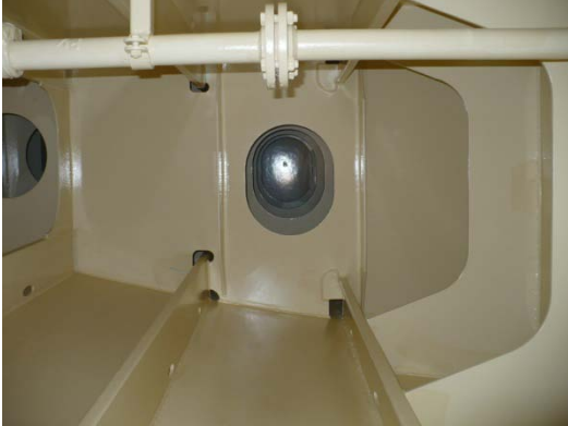
Double bottom ballast water tank (construction phase)
