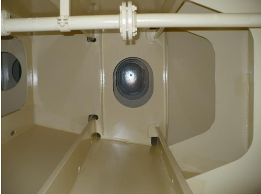
Double bottom ballast water tank (construction phase)
