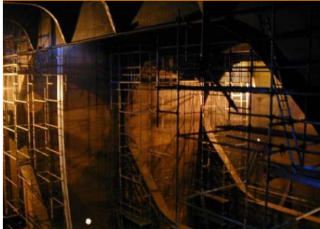
Scaffolding needed for the inspection of large cargo holds
